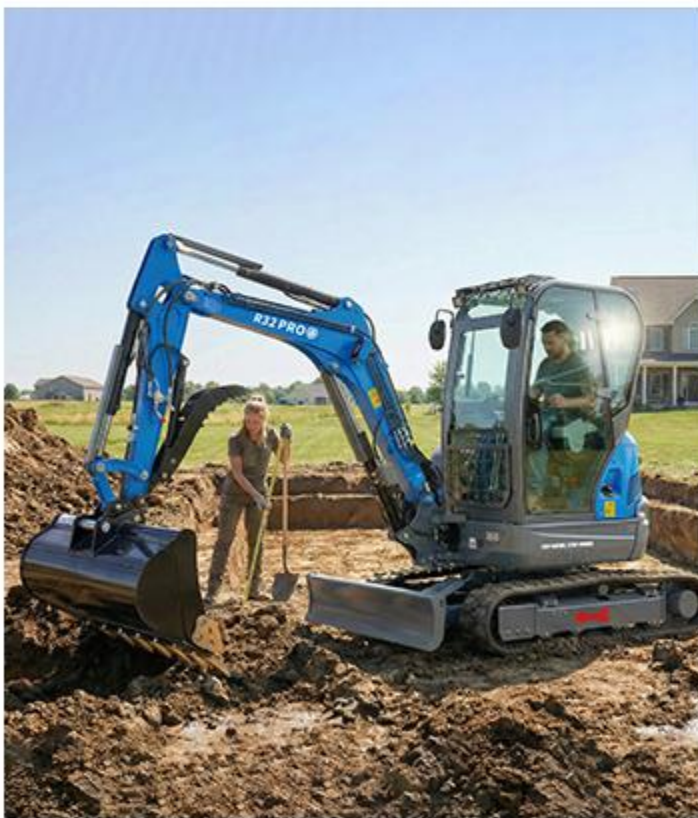
DIG A SWIMMING POOL
