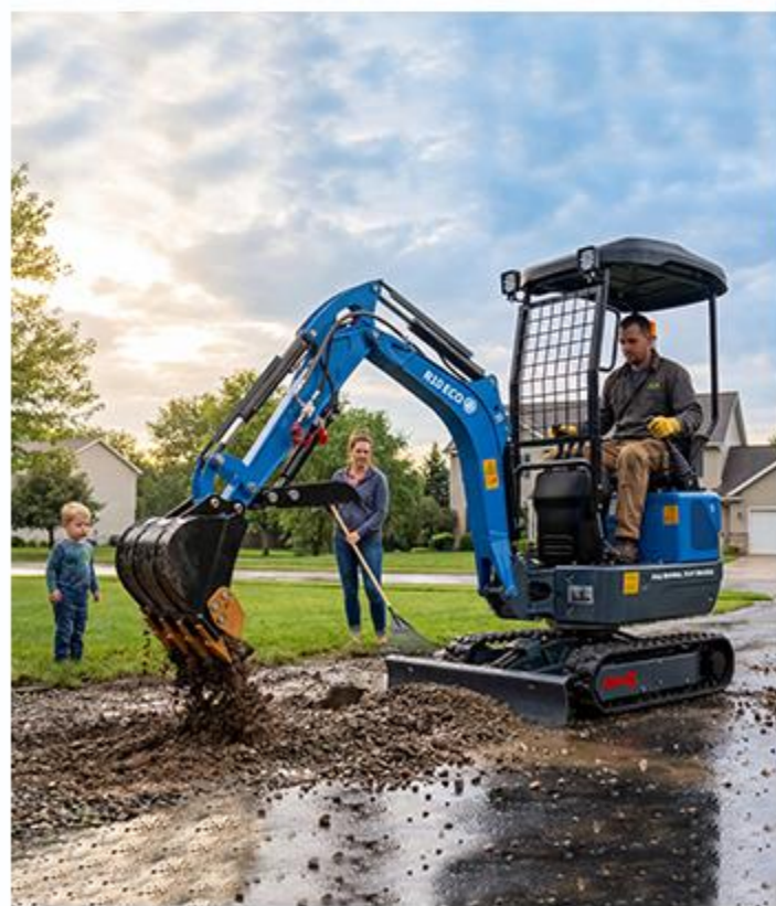
REPAIR A DRIVEWAY
