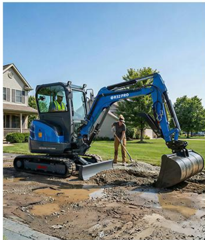
REPAIR A DRIVEWAY
