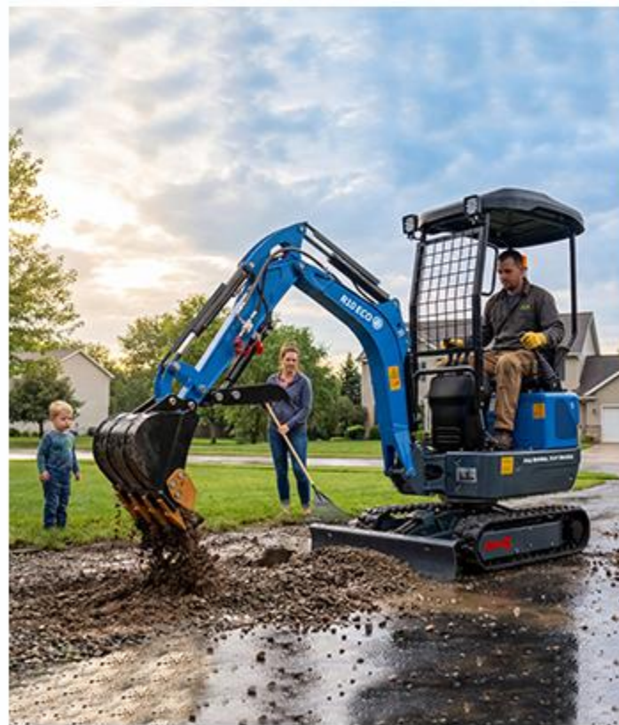
REPAIR A DRIVEWAY
